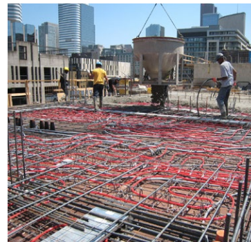
Radiant heating and cooling installation by REHAU at the YWCA Toronto Elm Centre. Image courtesy of REHAU.
