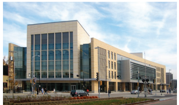
The Wisconsin Institutes for Discovery building at UW Madison features natural ventilation, a geoexchange system, aggressive heat recovery, and chilled beam technology, and is aiming to use 50% less energy and water than comparable facilities. Image: AEI.
