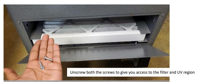
You may have to make some adjustments so that the access door is either completely off or fully open, like shown in the image
